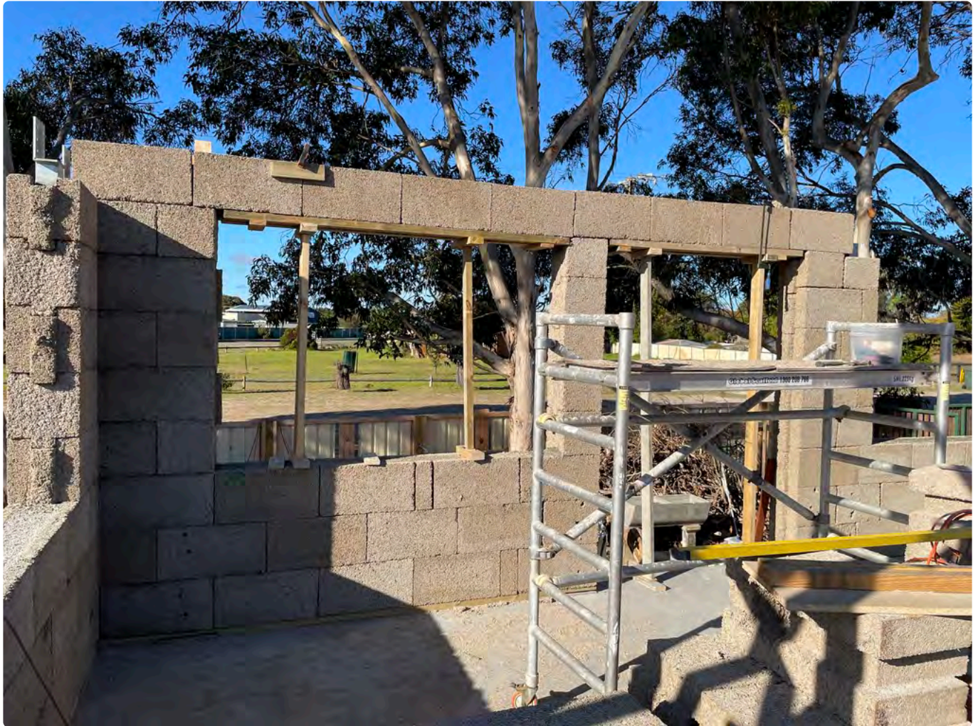
Timber lintel block supports.
